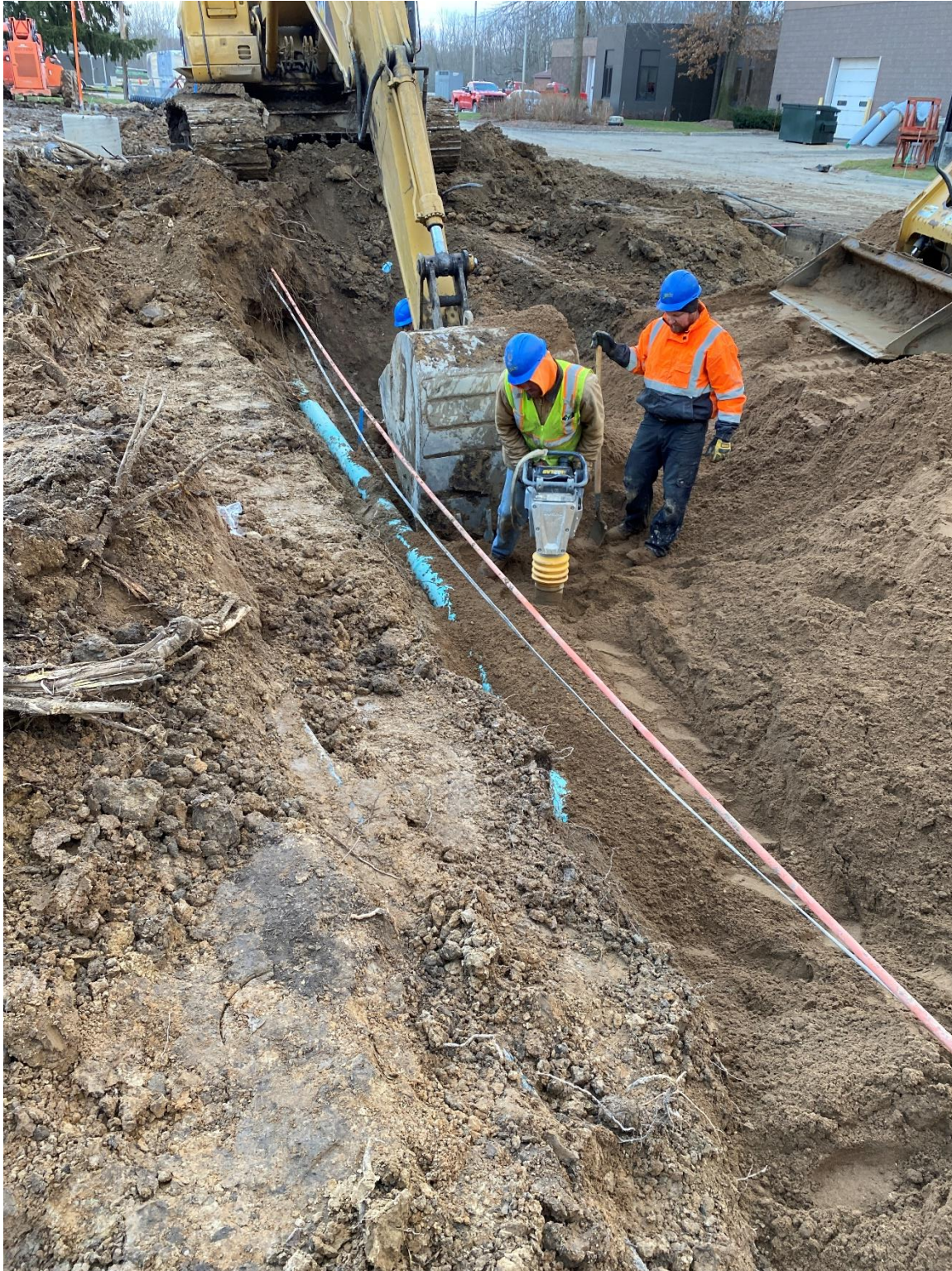
Watermain Installation and Backfill
