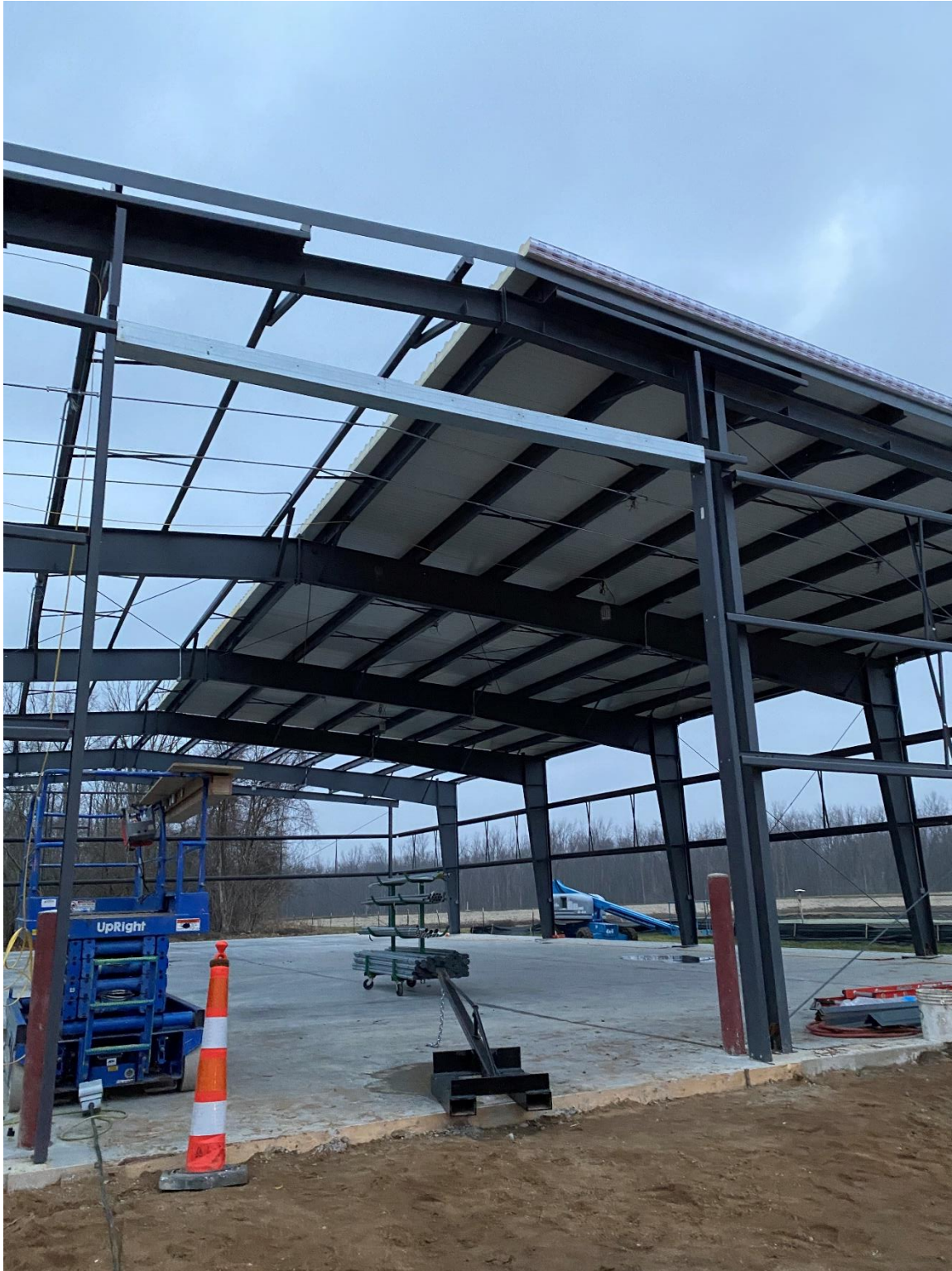
Maintenance Building Roof Panels Being Installed
