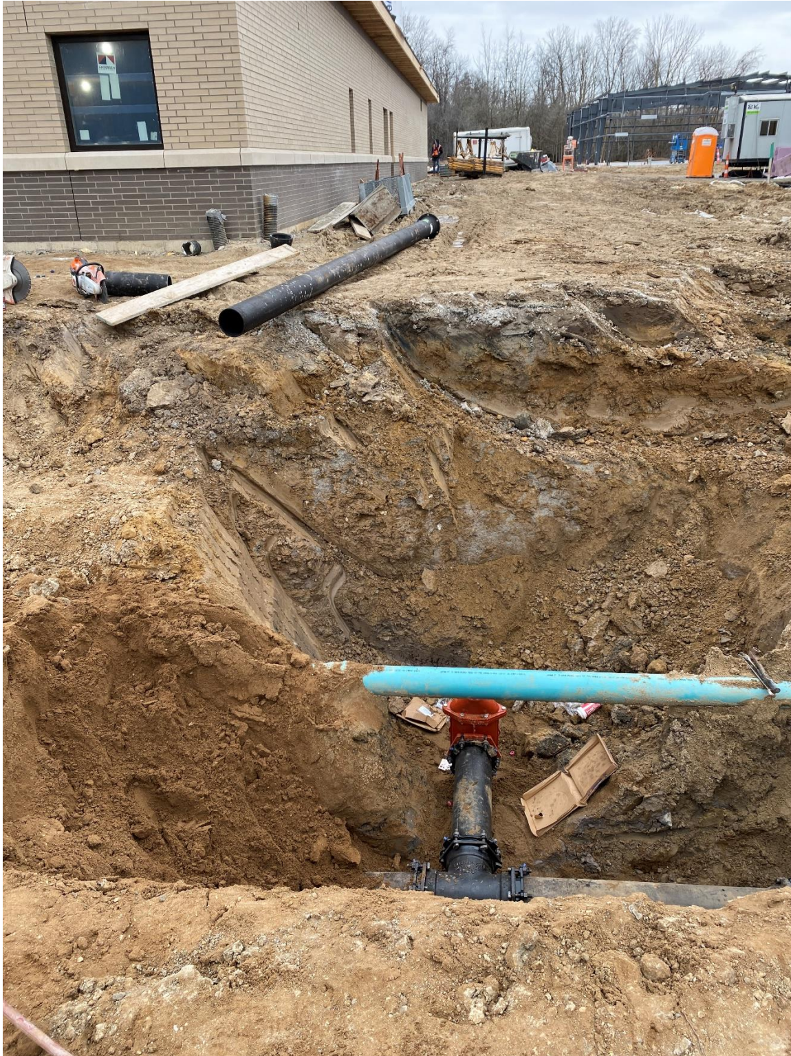
Watermain Installation Running North Along Administration Building
