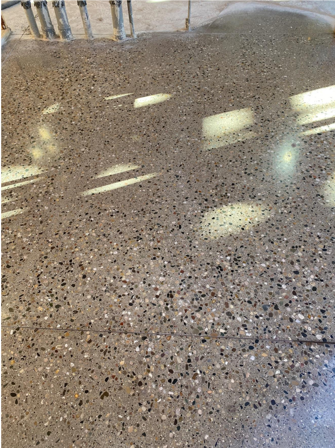
Polished Concrete Floor Sample Approval
